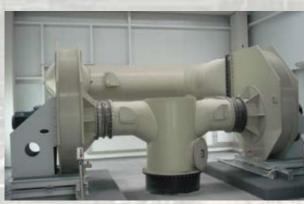
Deodorization Plant using Chemicals  $Q=35,000 \text{ m}^3/\text{h}$ .
