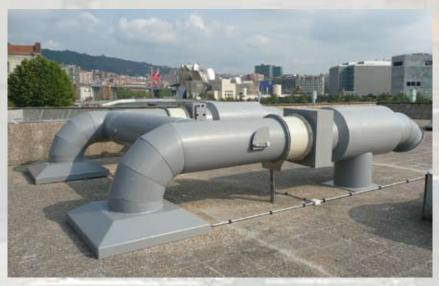
Deodorization and Ventilation Plant  $Q=18,100 \text{ m}^3/h$ .
