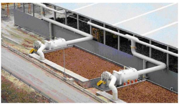
Biofiltration Deodorization Plant, Q=72,000 m³/h y Q=50,000 m³/h; RSU treatment plant.
